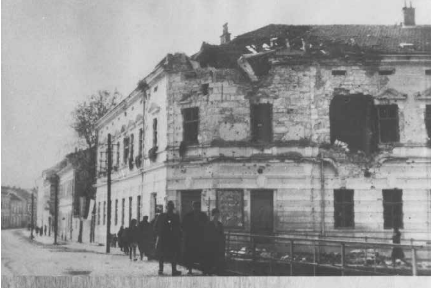
Fig. 3: Bihać, 4 November 1942. The photo shows the Kloster building, which was one of the last lines of Ustasha defence during the Partisan attack on the town. In the same building, the First Anti-Fascist Council for the National Liberation of Yugoslavia (AVNOJ) was held on 26 November 1942. (Courtesy of the Public Institution Museum of the Una-Sana Canton)
